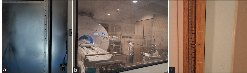
Figure 2: Photographs of (a) wall shielding, (b) screened window shielding, and (c) door shielding in the magnetic resonance scanner room.
